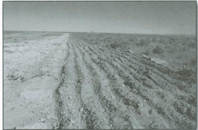
Figure 4—Rangeland drills produced deep furrows on these pipeline rights-of-way in Wyoming. The furrows help collect moisture and protect seedlings from wind.
